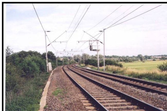
10 m between the stanchions here
